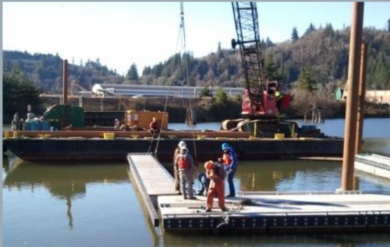
Installation of final finger float by Port staff and Billeter Marine.
