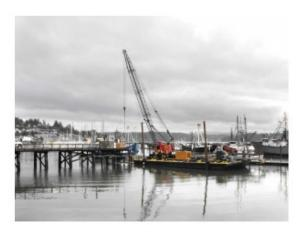
Crews working for Billeter Marine have been replacing piles at Port Dock 5 on Yaquina Bay this week to ensure safety and the provision of utilities and fuel to the adjacent floating docks. (Photo by Philip Swett)
